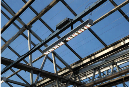
Pictured: A high-output and passively cooled LED fixture designed to replace an overhead HPS fixture. This fixture produces white light from a combination of blue, green and red wavelengths.
