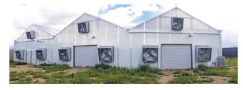
Pictured: By implementing the right cladding, growers can raise their structure's R-value and improve its heat retention, helping to reduce the operation's overall heating requirements.
