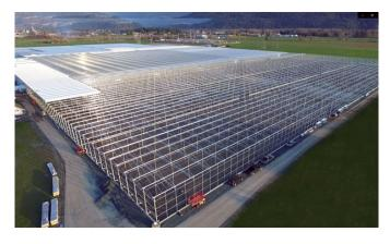
Pictured: Rainbow Green-houses is in the process of expanding at two locations. This one, which will be 10 acres, is at their site in Chilliwack, British Columbia. The inside will include new HPS lights, conveyers and ErfGoed flood floors.
