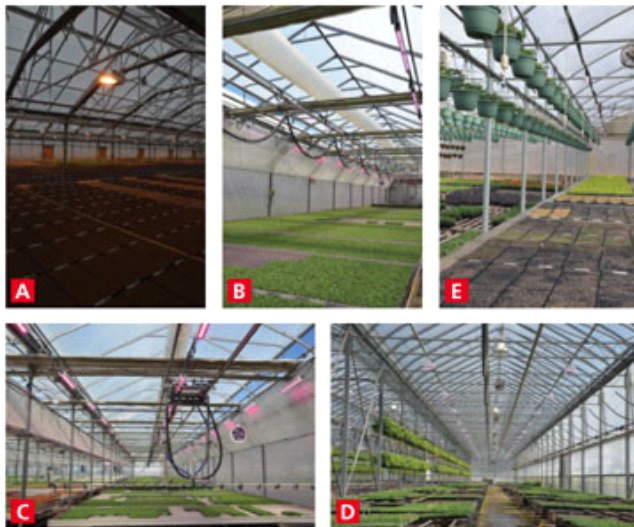
Figure 1. Supplemental lighting of young plants utilizing A) high-pressure sodium lamps, B-D) various commercially available high-intensity light emitting diode (LED) fixtures or E) LED photoperiodic lighting.
