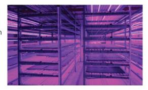
Seed needs a temperature controlled germination room to allow for some species to be germinated in a controlled climate when it would otherwise be too hot in the greenhouses. The new facility provides this, as well as a cooler for stratification of seed trays for hard-to-germinate seeds, daylength control and an in-house seed tray filler that allows for varying media mixes for specific seeds for even small batches.
