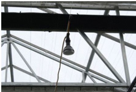
Figure 3. Light-emitting diodes (LEDs) are a new technology with great promise for use in photoperiodic lighting.
