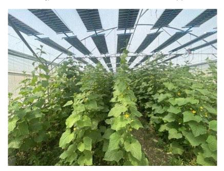
The initial prototype was built by one of the consortium's partners, TriSolar. The idea: to combine optimum crop conditions with significant energy production, including using agrivoltaics in areas with lower light conditions. Solar panels are mounted on a responsive tracking system in the greenhouse, with a controller that changes the angle of the panels according to the plants' needs. By using CO2 enrichment, they can increase plant growth while allowing for lower-light
