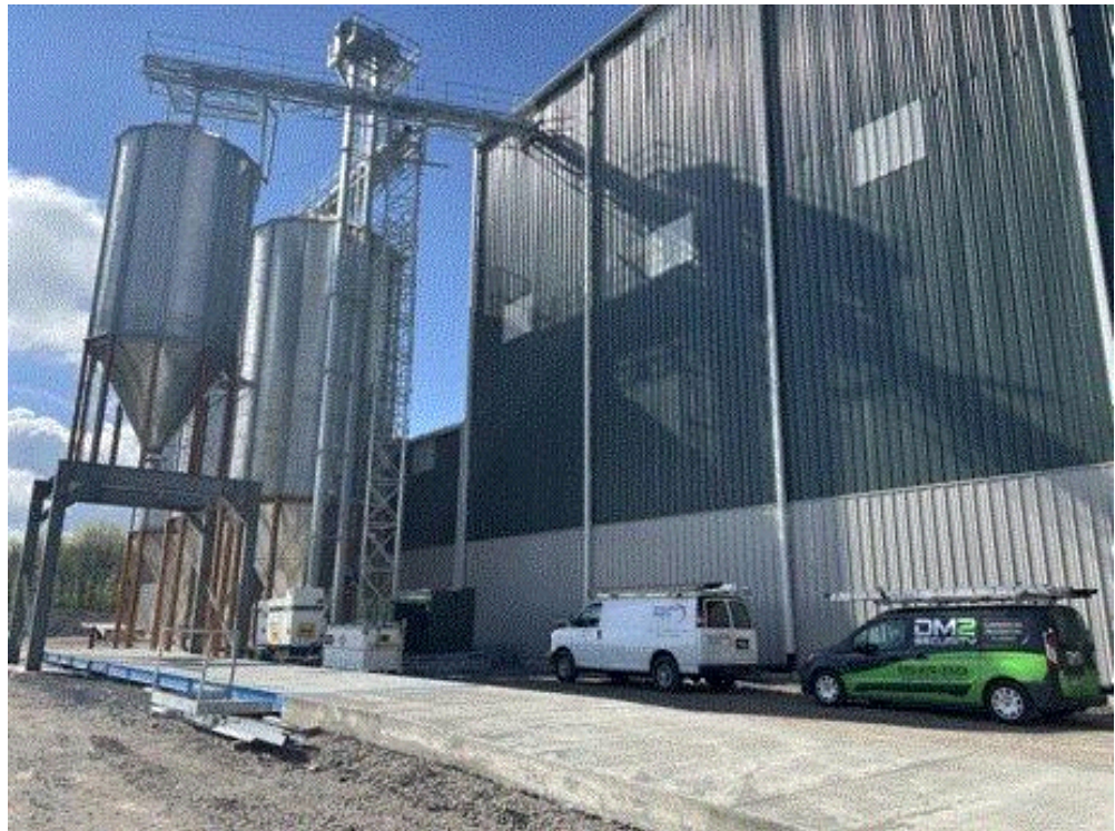
The silos on the outside of the facility, including one designed to load trucks from the top. There's a heavy duty scale built in to make sure the trucks are loaded accurately.
