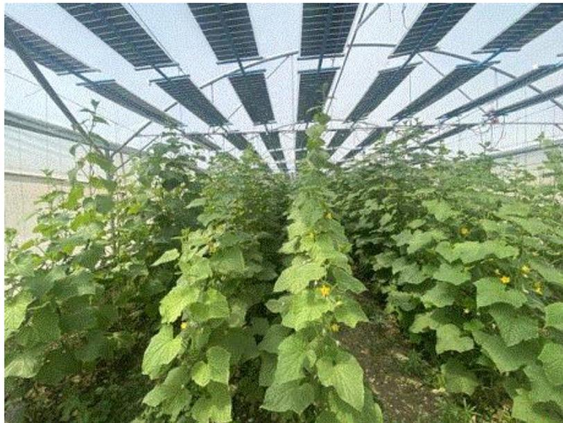
The initial prototype was built by one of the consortium's partners, TriSolar. The idea: to combine optimum crop conditions with significant energy production, including using agrivoltaics in areas with lower light conditions. Solar panels are mounted on a responsive tracking system in the greenhouse, with a controller that changes the angle of the panels according to the plants' needs. By using CO2 enrichment, they can increase plant growth while allowing for lower-light
