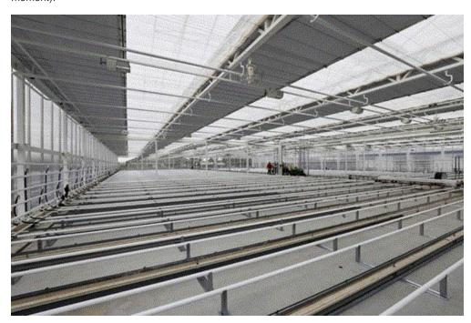
The greenhouse structure, which replaces a wood and glass structure from the '60s, is by Nobutec. Luiten supplied the three-layer curtain system: 50% shade on top, and an energy curtain and light pollution curtain below (to prevent night lighting from annoying the neighbors). Luiten is also installing horizontal curtains to divide the house into six growing zones.
