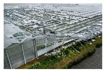
If you search online for "Dutch greenhouse collapse," you can find frightening security camera footage of the moment this giant glass tomato range collapsed, pushed by strong winds and weakened by workers who'd removed some structural beams to make room for a new curtain system.
