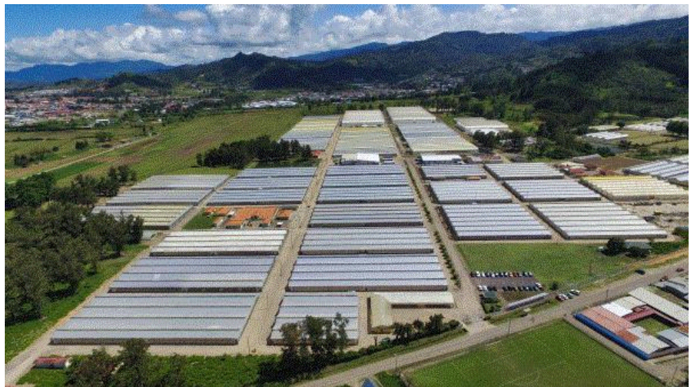
Linda Vista Farm 2. The Francis Kwong Center is the white roof, center right.
