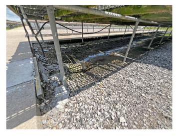
They've installed concrete culvers under each bench of the outdoor production area to help drain any flood waters that breach the levee (inset). All of the benches are now made of metal set in concrete instead of placed on cinder blocks. And they've been fitting all of their greenhouses with reinforced double poly that can withstand 100-mph winds.
