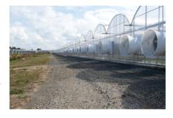
electricity when they're running. These fans get a lot of their efficiency from the fact that they have direct drive motors with frequency drives—there's no fan belt to maintain or replace. Yes, it came at a premium, but we figure a seven-year payback.
