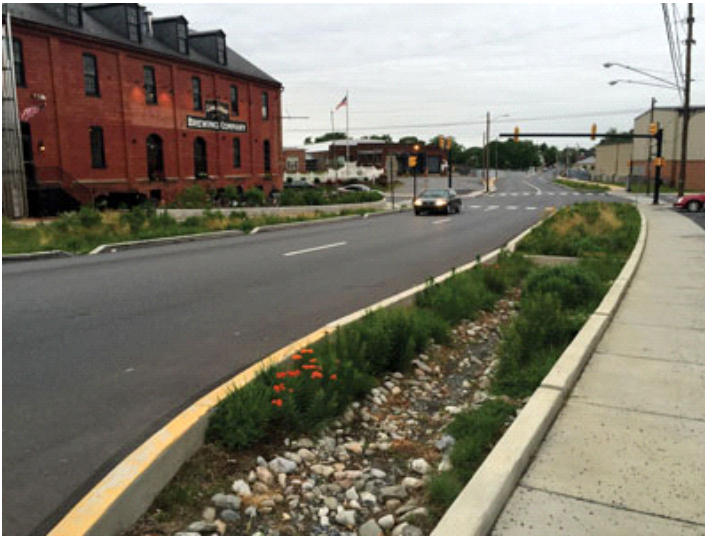
Pictured: Streetside stormwater green infrastructure at Lancaster Brewing in Pennsylvania. North Creek Nursery's Claudia West redesigned the planting plans after the engineers were having problems. This photo from June 2015 shows plants the first season after replanting.
