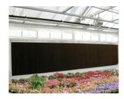
Systems come complete with Kuul Pads, top and bottom aluminum distribution, end panels, sump pump and plumbing kit.
