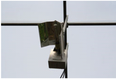
Figure 2. A high-pressure sodium (HPS) lamp with an oscillating reflector is a newer technology used to provide photoperiodic, not supplemental, lighting to plants in the greenhouse.
